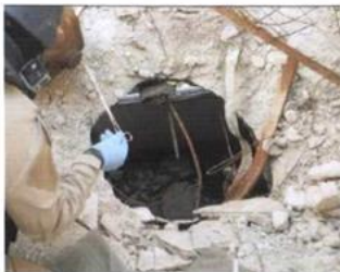
The shape and dimensions of the resulting aperture are consistent with the penetration of a solid body through the reinforced concrete barrier under the angle of 80-90 °
