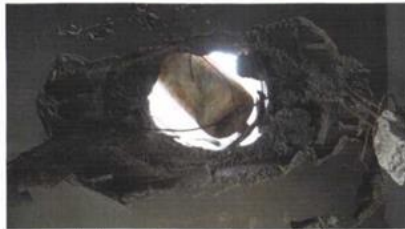
Black scorching on the crater and the destruction of steel rebar inside the aperture
