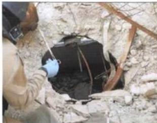
The shape and dimensions of the resulting aperture are consistent with the penetration of a solid body through the reinforced concrete barrier under the angle of 80-90 °
