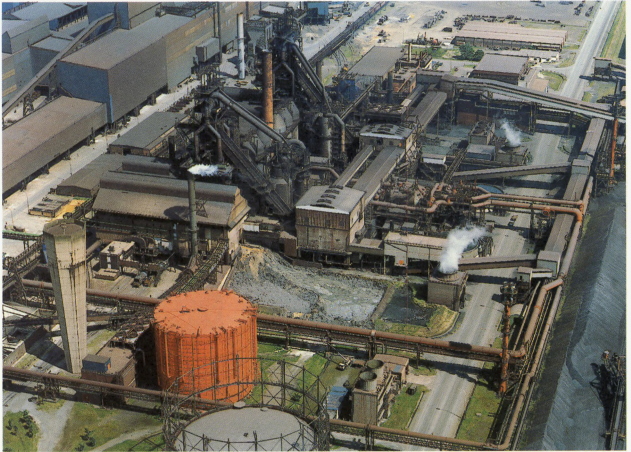
Photo 6: Aerial view of blast furnaces with slag pits and gas holders in foreground
