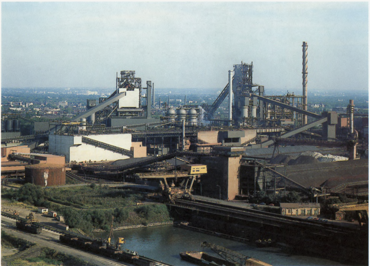
Photo 4: Two large modern blast furnaces with raw material stockpiles in foreground
