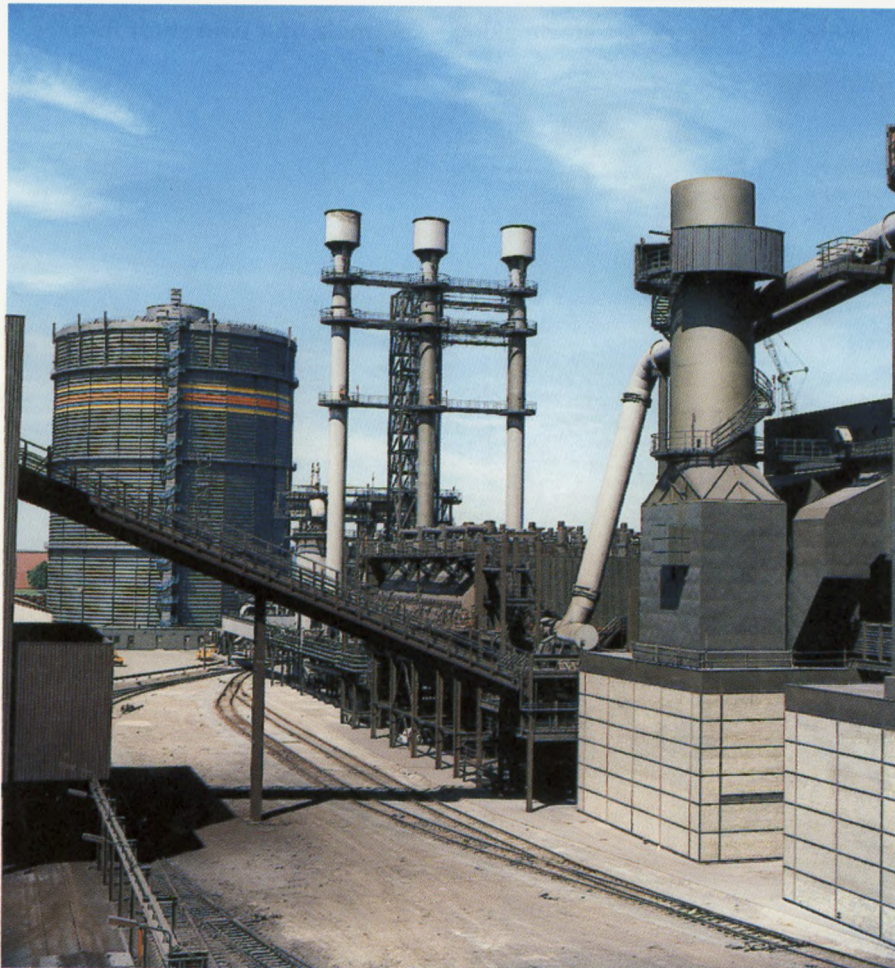
Photo 13: Gas recovery plant at a BOS plant
