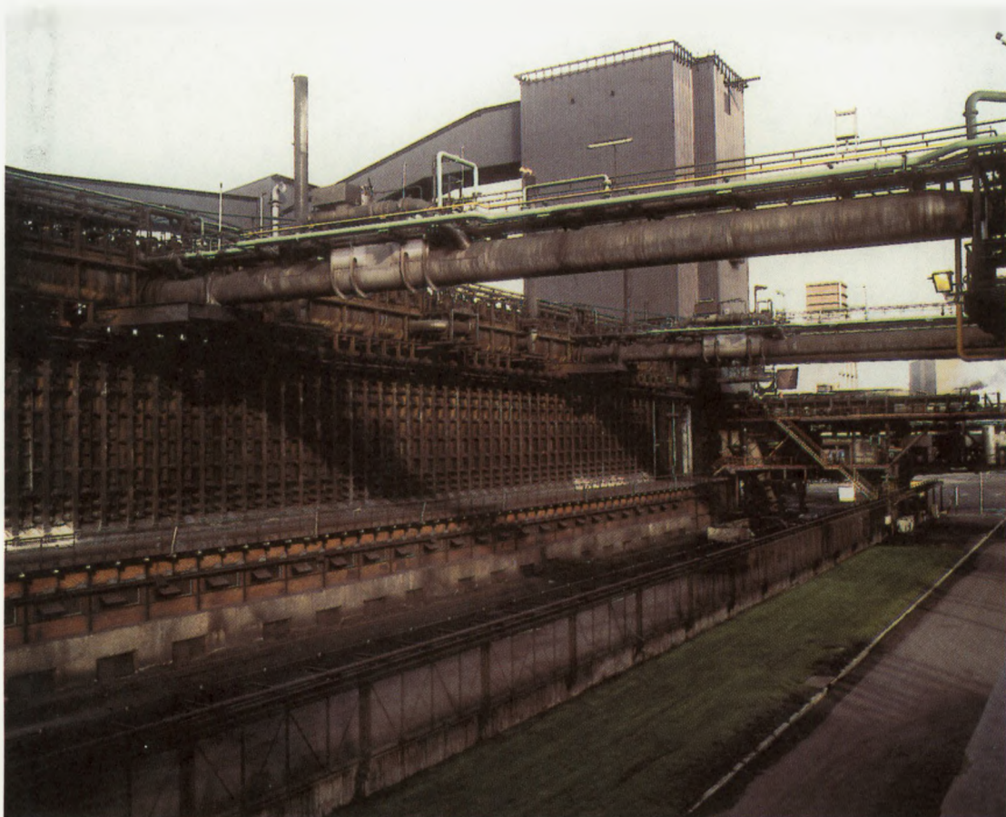
Photo 5: A coke oven battery
