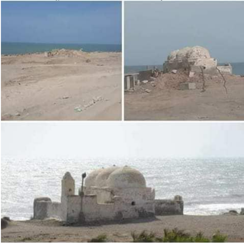
Figure 42.2 Picture showing the destruction of the Mosque 166
