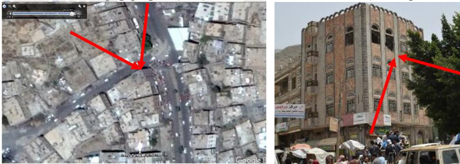
Figure 35.D.1 Location of building targeted at (13°34'9.51"N, 44° 0'0.01"E) with potential direction of attack
