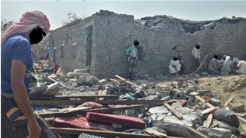
Figure 33.B.1 Pictures showing damage to the house and tent 73
