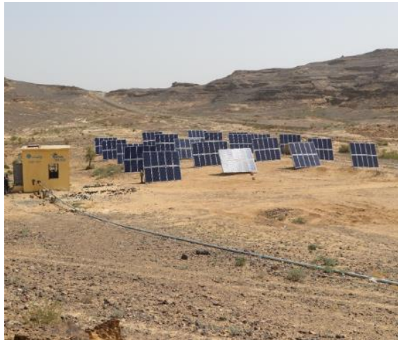
Figure 33.D.2 Site before the attack
