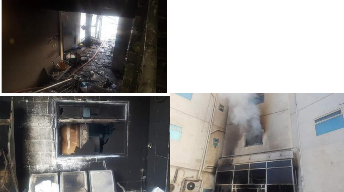
Figure 37.1 Damage to the hospital 149
