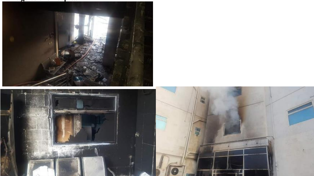
Figure 37.1 Damage to the hospital 149
