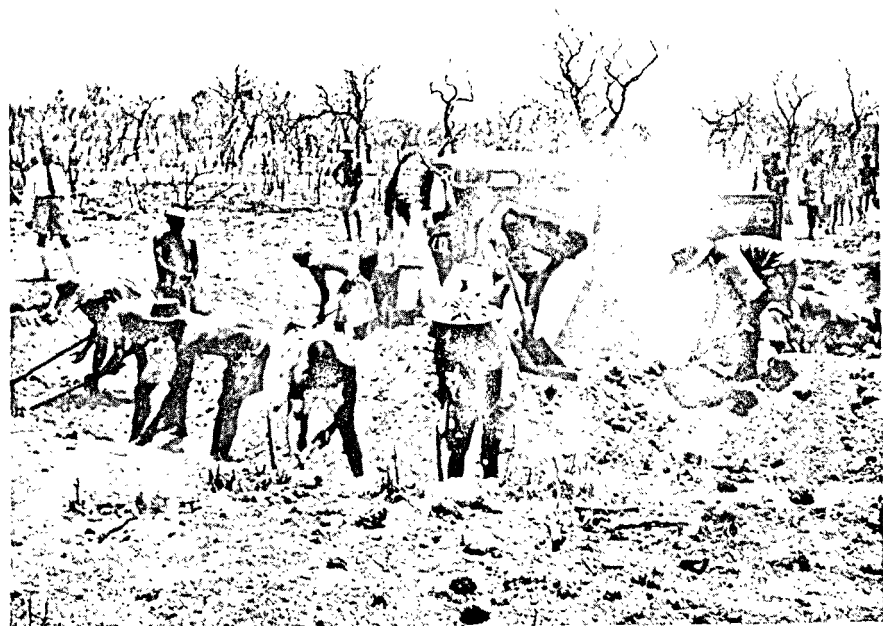
Work on the new Yendi-Nalerigu road
