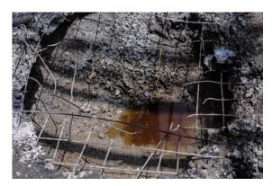
Figure A.60.6 **Damage at impact point of EO**
