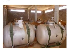
Figure D.36.12 Liquid bi-propellant oxidiser field storage tank<sup>35</sup>
