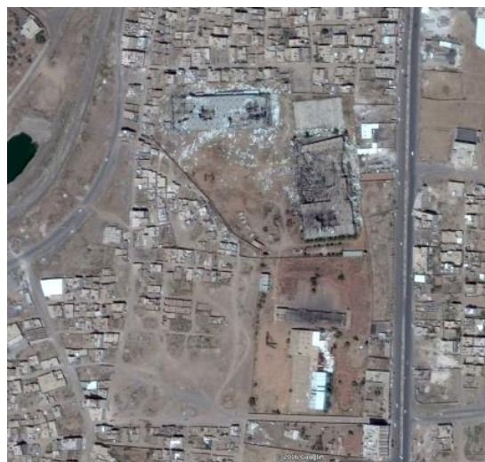
Figure C.60.2 Alsonidar complex (3 October 2016) post attack
