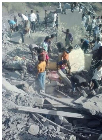
Figure E.60.2 Post blast damage
