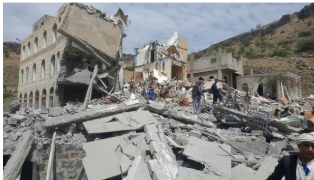
Figure B.58.4 Post-blast damage
