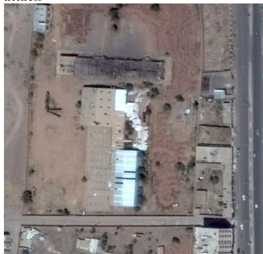
Figure C.60.4 Red Brick factory (3 October 2016) post attack
