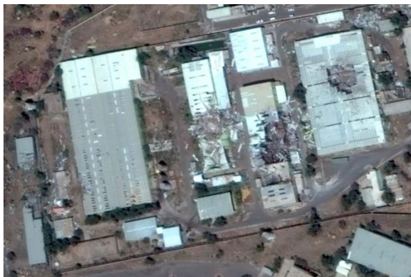
Figure A.60.4 Second strike damage (Post August 2016)
