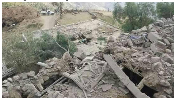
Figure C.58.4 Damage to al-Maqadhi houses (second strike)
