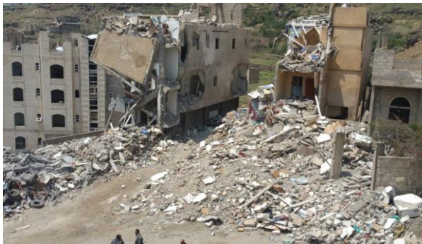
Figure B.58.2 Post-blast damage
