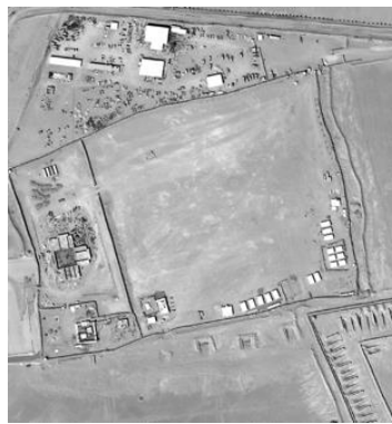
Figure 65.2 Bir Ahmed detention location (07 November 2017) 22
