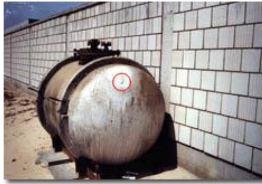
Figure D.36.12 Liquid bi-propellant oxidiser field storage tank 35
