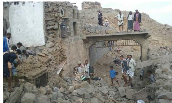
Figure C.58.5 Damage to al-Maqadhi houses
