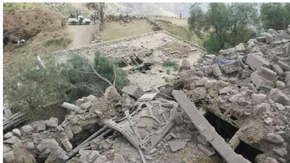
Figure C.58.4 Damage to al-Maqadhi houses (second strike)
