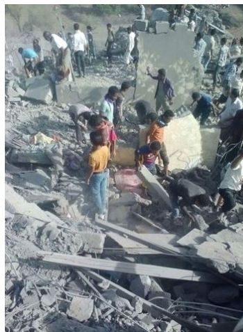
Figure E.60.2 Post blast damage
