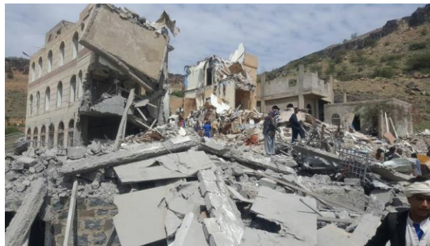
Figure B.58.4 Post-blast damage
