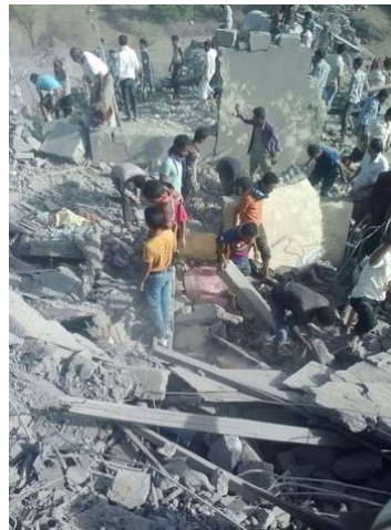
Figure E.60.2 Post blast damage
