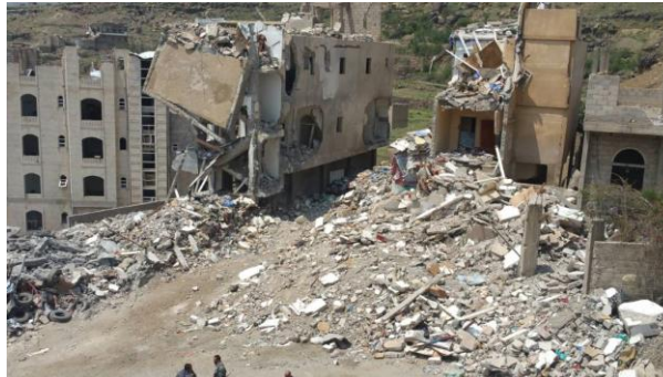
Figure B.58.2 Post-blast damage
