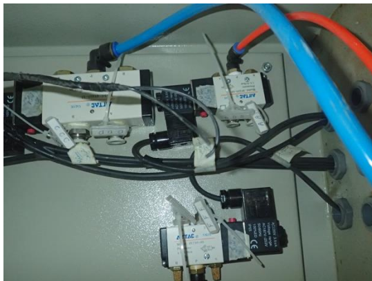
Figure D.36.24 Solenoid Valves Models 4V210-08 / 4V110-15 (Partial Traced: > IR)
