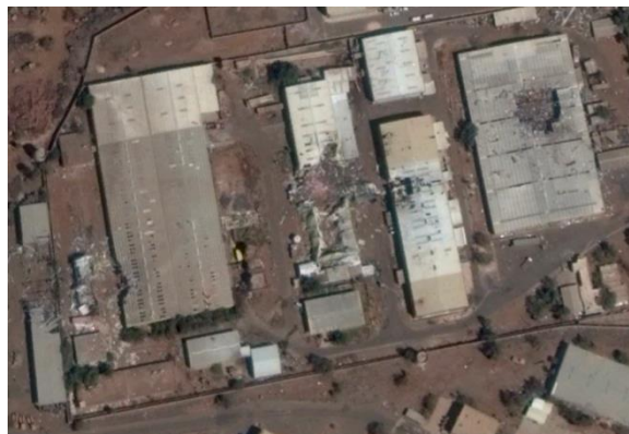
Figure A.60.3 First strike damage (29 February 2016)
