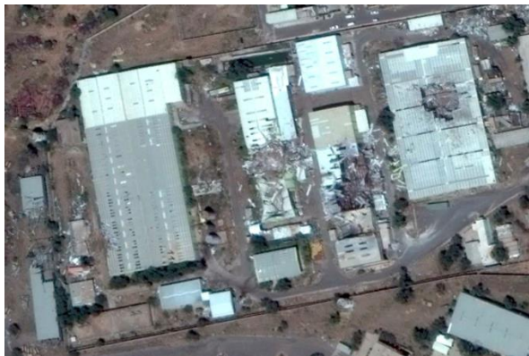
Figure A.60.4 Second strike damage (Post August 2016)
