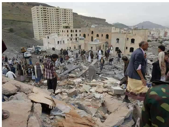
Figure B.58.1 Post-blast damage 72
