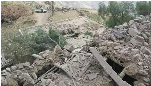
Figure C.58.4 Damage to al-Maqadhi houses (second strike)
