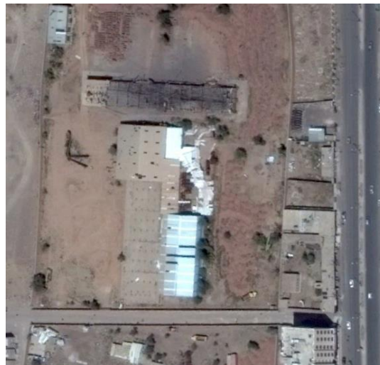
Figure C.60.4 Red Brick factory (3 October 2016) post attack
