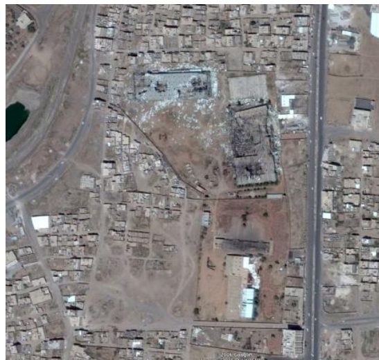
Figure C.60.2 Alsonidar complex (3 October 2016) post attack
