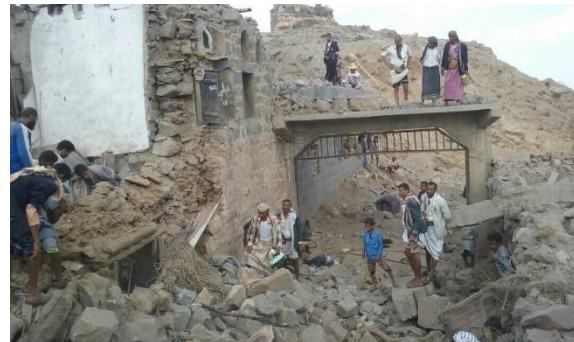
Figure C.58.5 Damage to al-Maqadhi houses
