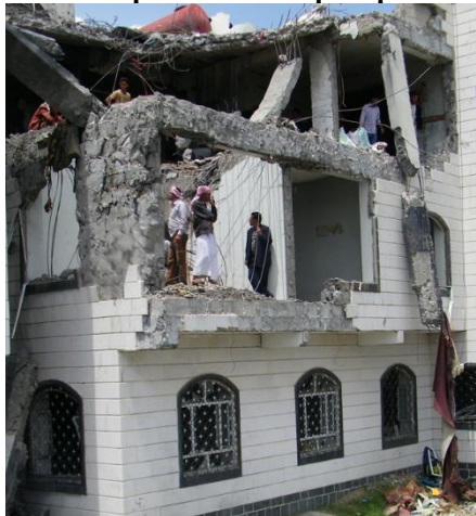
Figure D.60.4 Civilian apartment complex post blast
