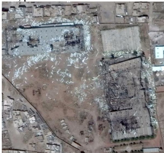
Figure C.60.3 Steel and Water Pumps Factories (3 October 2016) post attack
