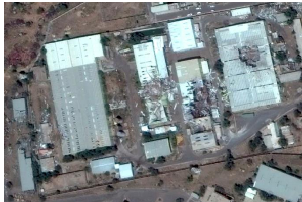
Figure A.60.4 Second strike damage (Post August 2016)
