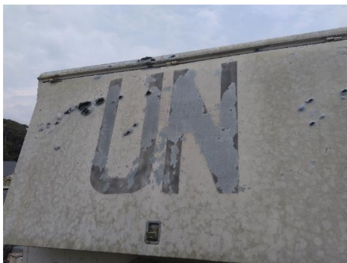
Bullets' impacts on the UN mobile water treatment unit
