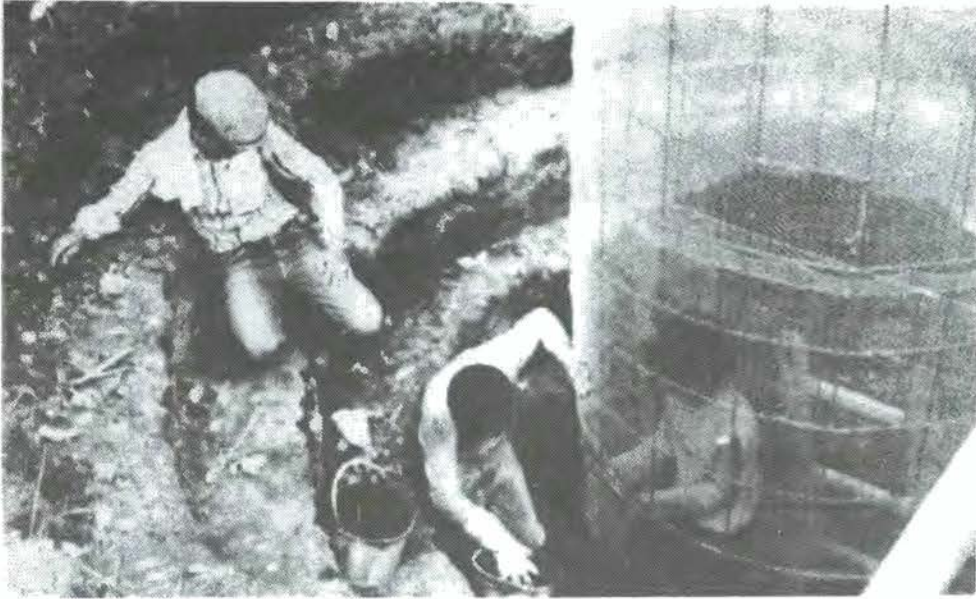
Fig.5.6 Plastering of digester frame
