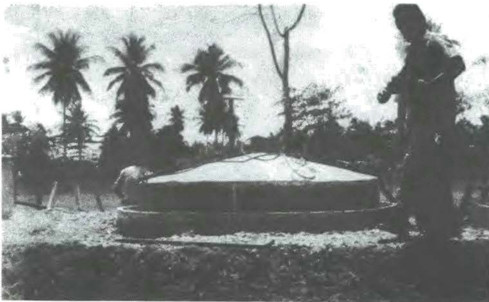
Fig.5.9 Gas holder in place
