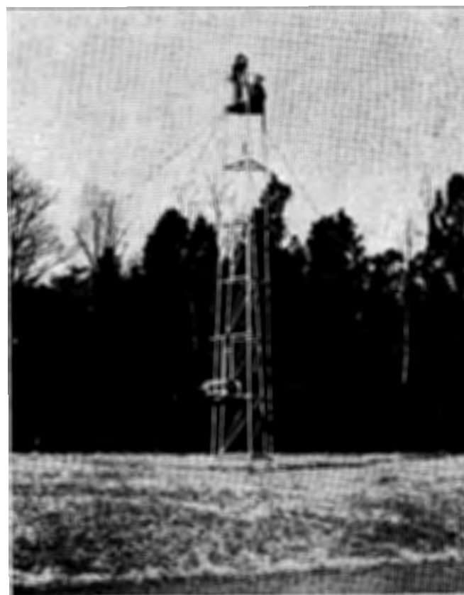
Figure 23. Fieldmen using theodolite on portable tower
