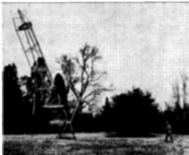
Figure 21. Erecting portable surveying tower
