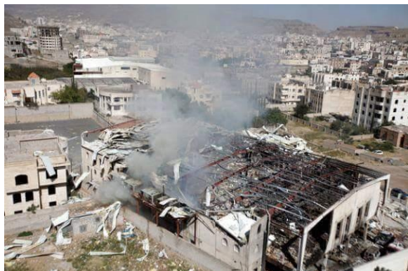
Figure 49.D.2 Post blast aerial image 298
