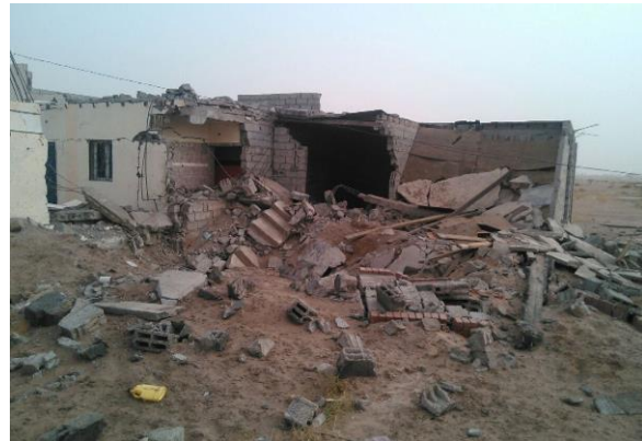
Figure 49.B.3 Armed group suspect's house post-explosion
