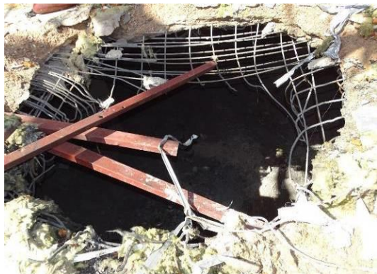
Figure 49.D.4 Entry point EO1
