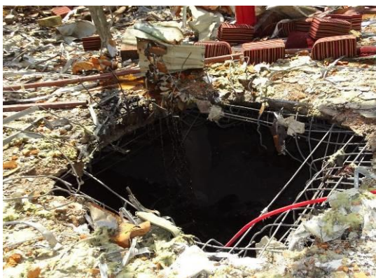
Figure 49.D.5 Entry point EO 2
