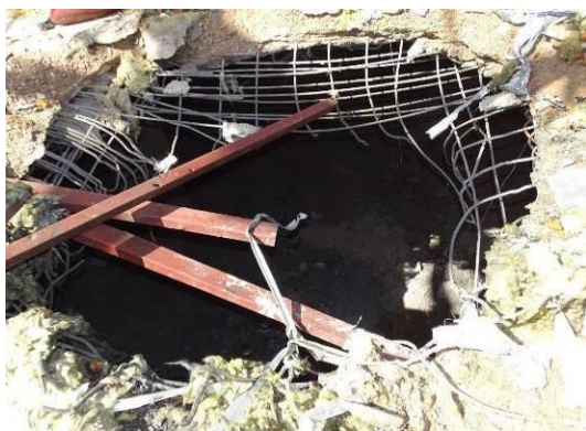
Figure 49.D.4 Entry point EO1
