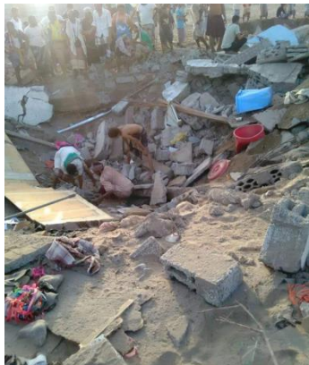
Figure 49.B.2 Civilian house post-explosion 243
