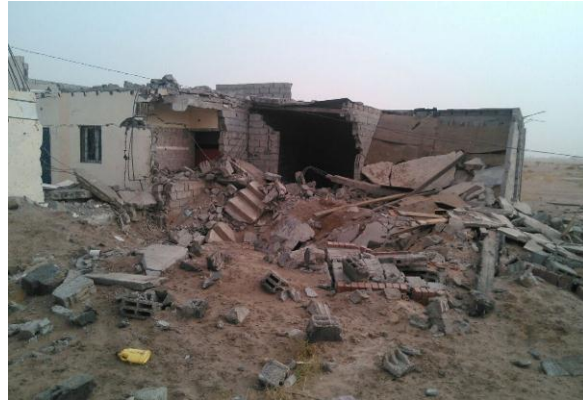
Figure 49.B.3 Armed group suspect's house post-explosion
