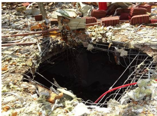
Figure 49.D.5 Entry point EO 2
