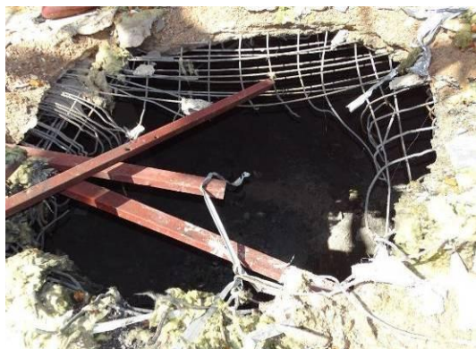
Figure 49.D.4 Entry point EO1
