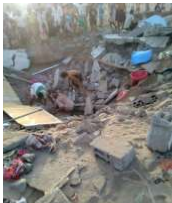
Figure 49.B.2 Civilian house post-explosion 243
