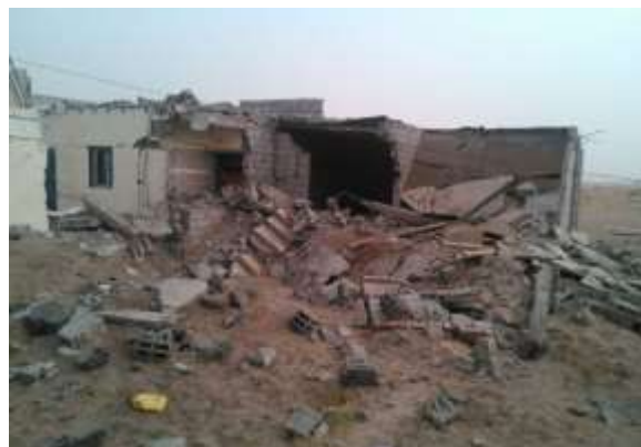
Figure 49.B.3 Armed group suspect's house post-explosion
