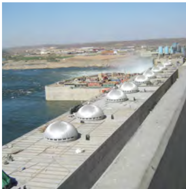
Merowe Dam, Sudan, 2009. Source: Ihab Jnad.
